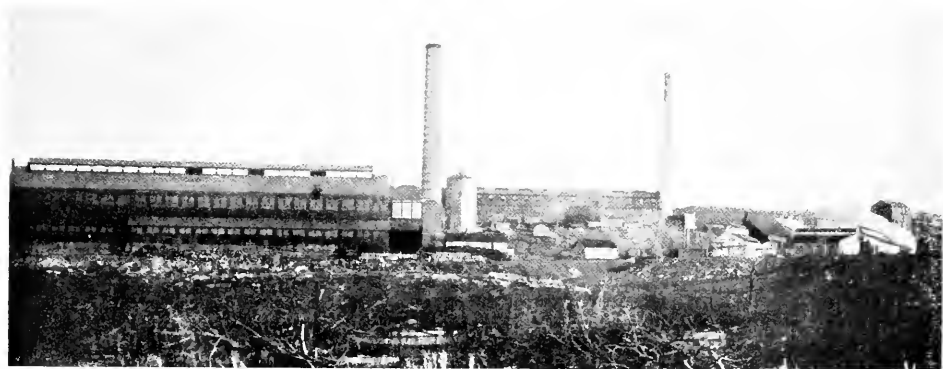
Fig. 77—General View of Coniston Plant, 1914, Mond Nickel Company, Ontario.
